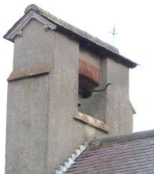
Top: Chancel, south slope. Above: Flashings to the bellcote with possible missing soakers. Below: View of the bellcote.
