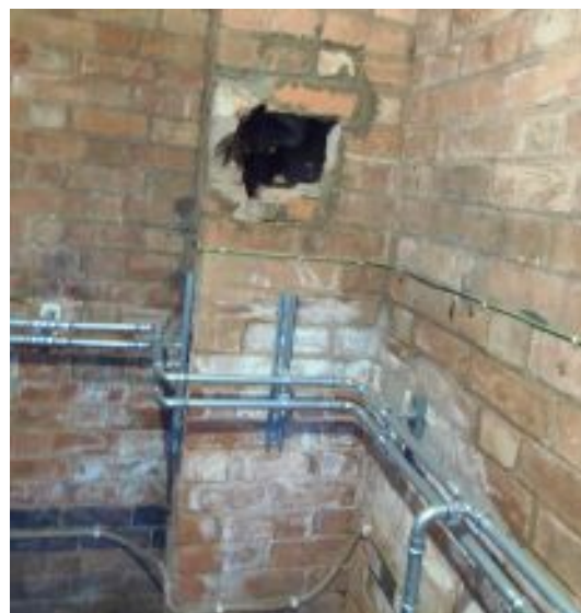
Above: Clergy vestry south wall, door through to the chancel. Below: Boiler room wall with cavity and un-insulated pipework. Bottom: Boiler room door.
