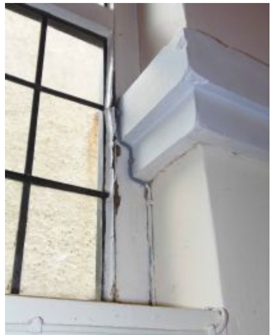
Above: Putty failing to the east window frame in the chancel. Below: View of the chancel, east wall. Second below: Chancel, south wall. Bottom: Nave north wall, 2nd bay from west.
