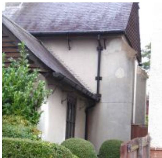
Above: Guttering and downpipe to the chancel south roof slope. Below: Guttering and downpipe to the boiler room east roof slope. Second below: Link to the hall flat roof and guttering. Bottom: Nave north slope guttering and downpipe to the west of the clergy vestry.
