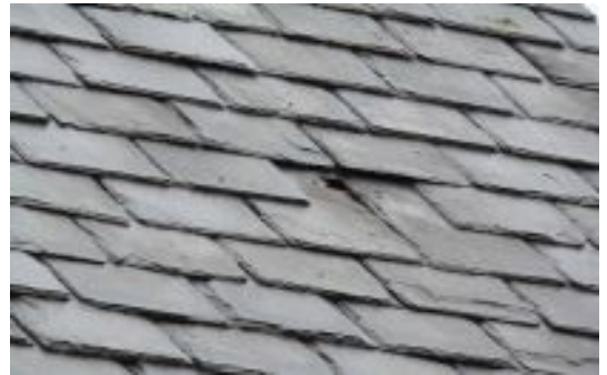
Top: Nave, north slope. Above: Missing slate to the western end of the nave north slope. Below: Nave, south slope. Second below: View of the choir vestry and roof. Bottom: East slope of the choir vestry roof and guttering.
