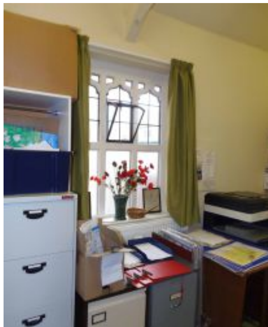
Above: Choir vestry east wall. Below: External door in the choir vestry west wall with some redecoration needed.
