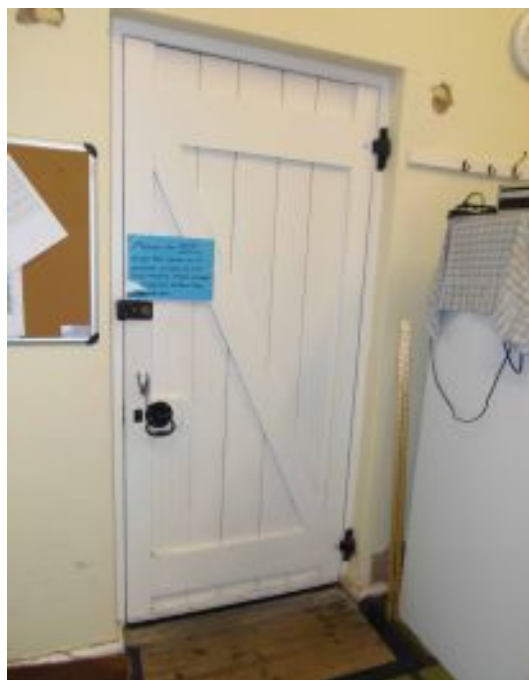
Bottom: Clergy vestry, north wall with water tank at high level.
