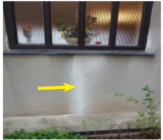
Above: Slight crack below the window in the 5th bay of the nave south elevation. Below: Choir vestry, west elevation. Second below: Crack above the window in the choir vestry east elevation. Bottom: View of the timber south porch.
