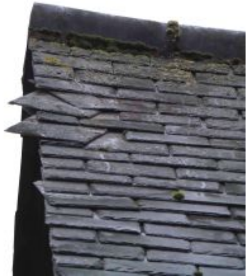
Above: Displaced slates to the east end of the chancel north slope. Below: Clergy vestry/boiler room, east slope. Second below: Displaced slates to the north east corner eaves. Bottom: Clergy vestry, west slope and valley gutter.
