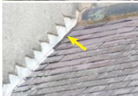
Top: Chancel, south slope. Above: Flashings to the bellcote with possible missing soakers. Below: View of the bellcote.
